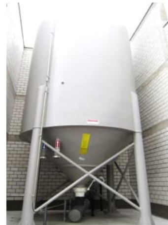
Pellet-Silo, 90 m3 Inhalt, H-13m
