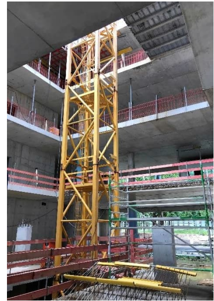
Blick in das Atrium
